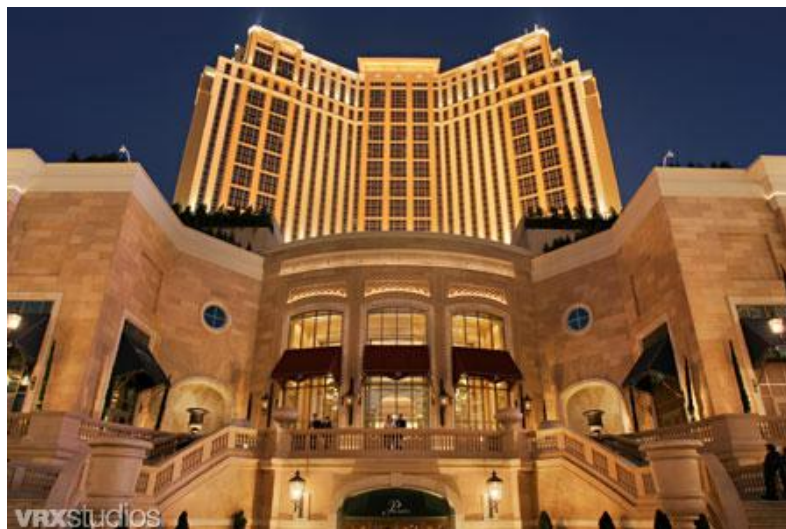
The Palazzo Resort Hotel & Casino, Las Vegas, NV
